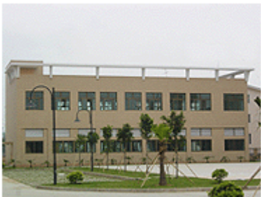
ETO Sterilization Room and Lab Center
